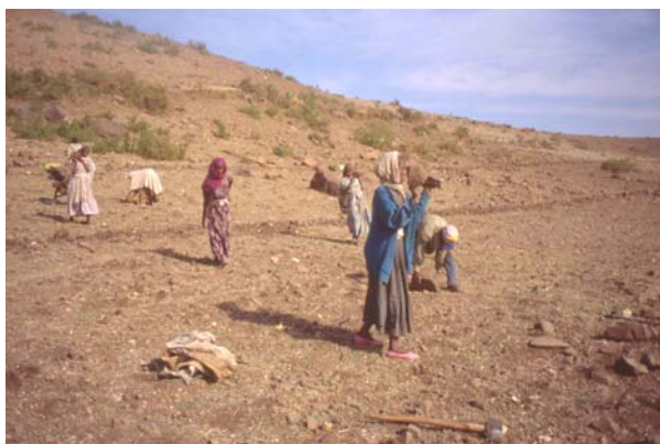
Figure 7. Stone collection for stone bund building (After Nyssen et al., 2001)
