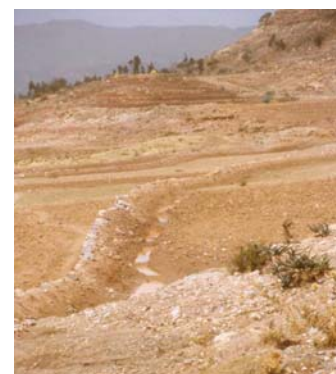
Figure 10. The building of stone faced trenches, i.e. stone bunds along tied ridges, allows the use of stone rich soil as backfill for the stone bunds and enhances infiltration.
